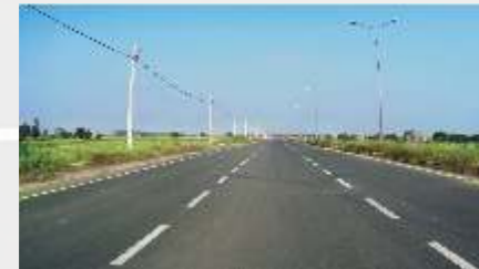
75M ROAD AND SECTOR ROADS READY
