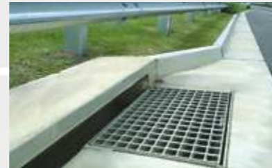
STORM WATER DRAINAGE & SEWERAGE LAID
