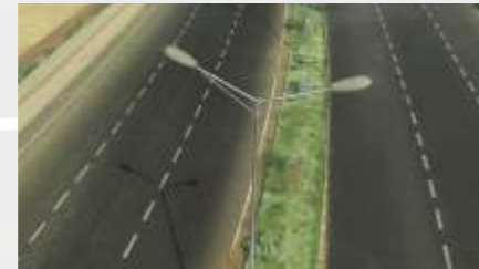
STREET LIGHTS INSTALLED
